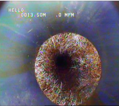
Development by bad sealing and use non-standard material may can leakage and contamination.
