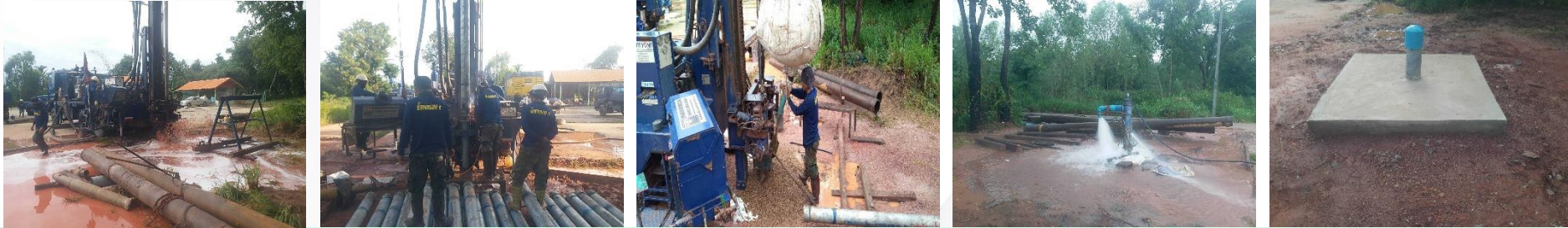
Drilling and develop groundwater wells
