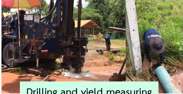
Drilling and yield measuring
